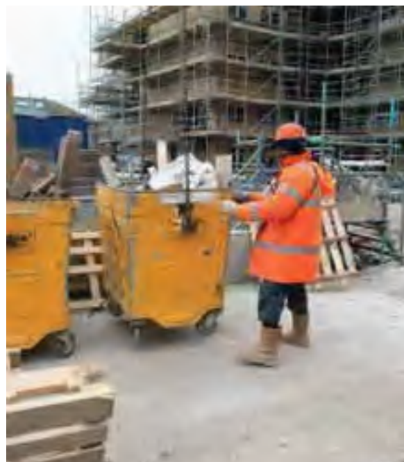
On-site separation of construction waste. Credit: WRAP
